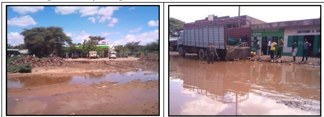
Figure 3.5.4: Ponding due to lack of drainage on main town streets.
